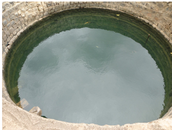
WATER LEVEL IN PWS WELL CHINCHOLI
